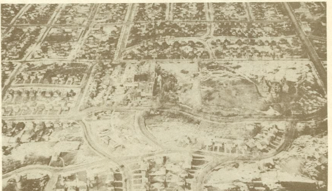
Washburn High School is under construction on the left; the Washburn Orphanage is on the right. Also visible is the expanding Washburn Park neighborhood, 1925, surrounding the site. (Minneapolis Board of Education)
